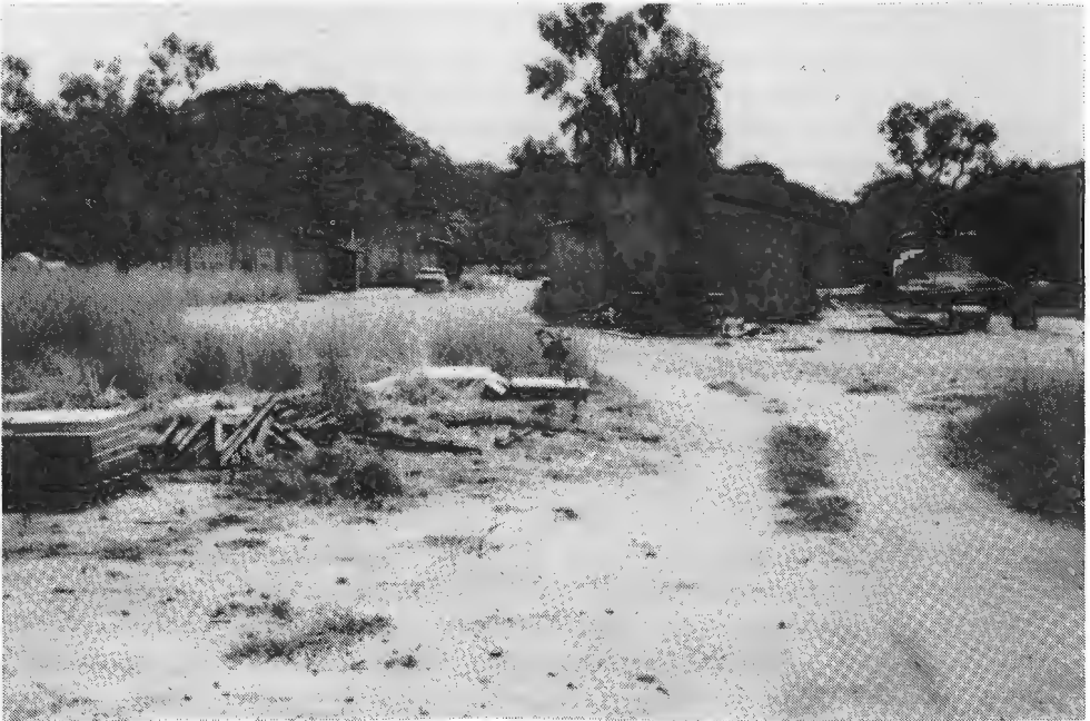
2. Construction of Looma settlement, 1975/6. The boulders on the ridge above represent Luma's children
