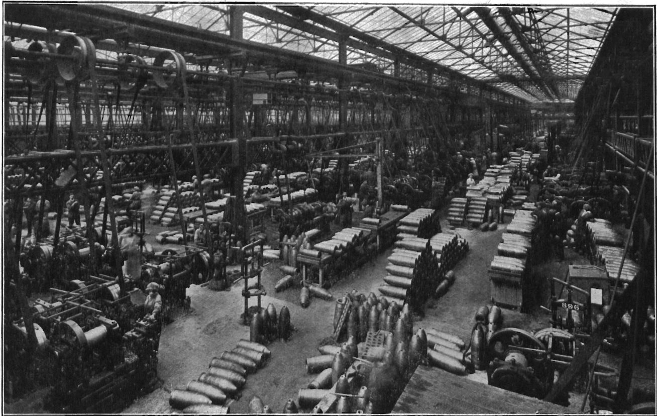
No. 36.—9,2 H.E. Shell Shop. General view of third bay.
