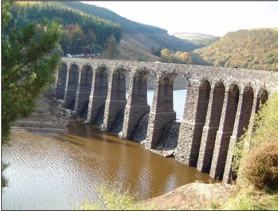
Figure 2 Garreg Ddu Combined Viaduct and 'Submersed dam'. Source: Geolocation (2013). ©Colin Price
