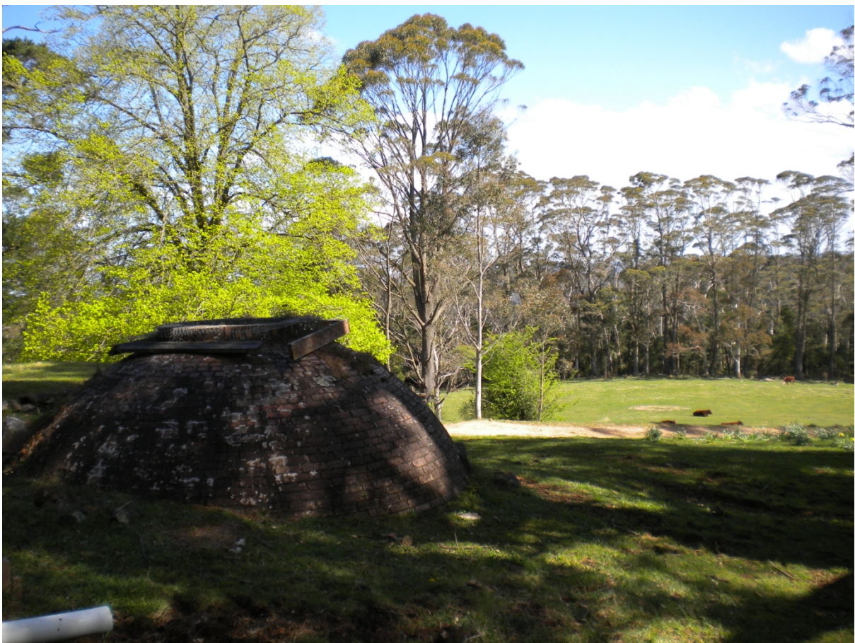
Cistern at Wynstay
