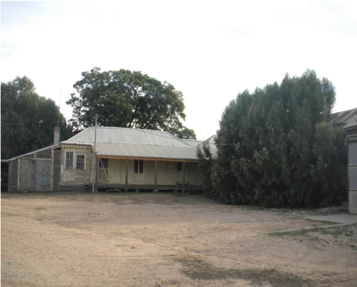
Accommodation outbuildings on Yanga station, March 2012
