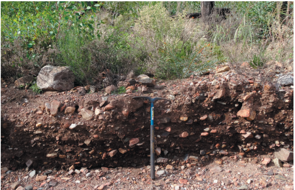
Figure 4. Debris flow levee material at levee 3 site.
