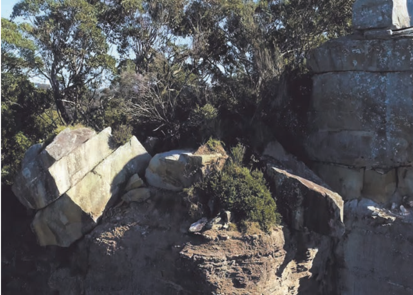
Figure 40. Large blocks of Hawkesbury Sandstone perched in the cliff top and resting on unstable shale. The three precariously stacked blocks on the left have a total volume of about 70 m 3 and weigh about 175 tonnes.
