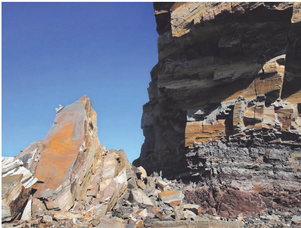
Figure 36. Large volume rockfall on Turimetta Head with extensive cracking in the face. Bald Hill Claystone and Garie Formation are 8 m thick at the base of the cliff.
