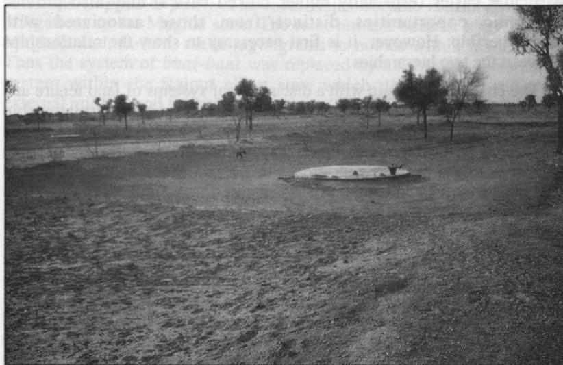
Photo 15: A private underground tank, with concave surface for collection of rainwater.
