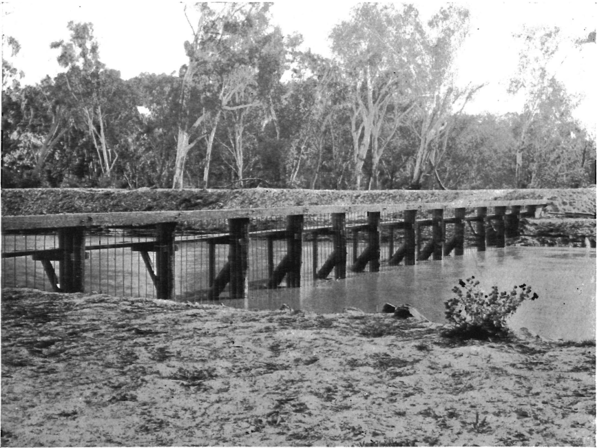
KOW SWAMP WORKS: DIVERSION CHANNEL FROM THE MURRAY.
