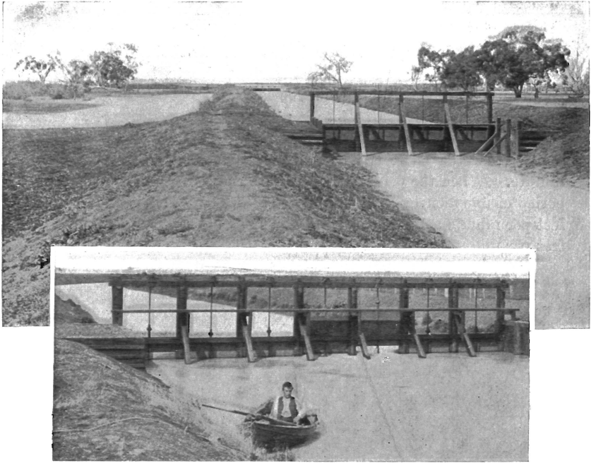
KOW SWAMP NATIONAL WORKS: MACORNA CHANNEL AND REGULATOR, VIC.
