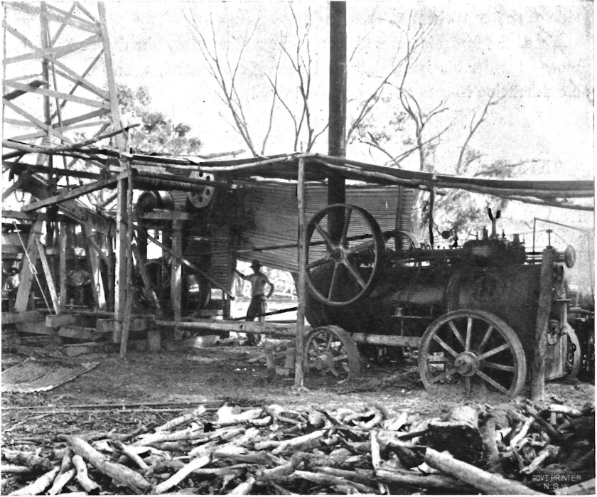
WINDING GEAR FOR HANDLING MUD PUMP AND HEAVY WORK.
