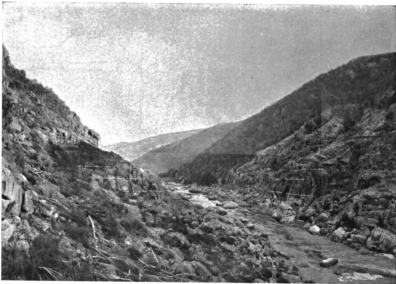
SITE OF BARREN JACK DAM WALL.
