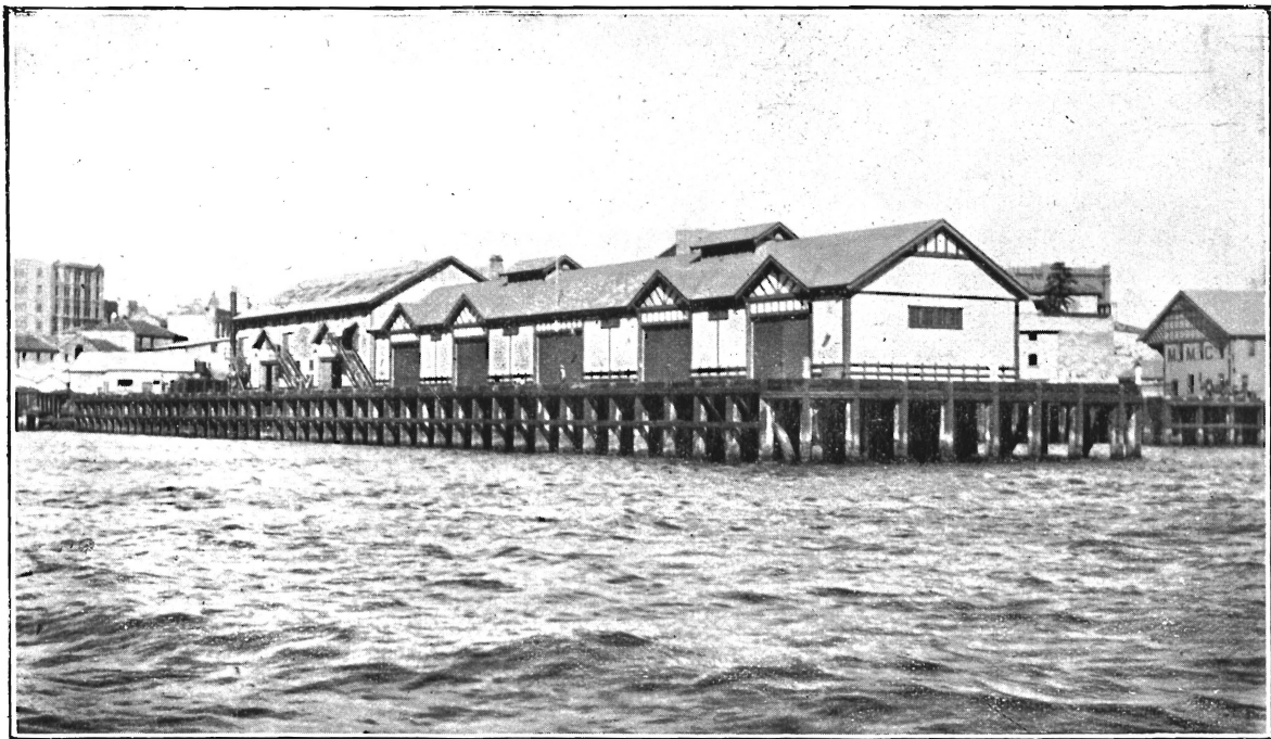
TYSER'S WHARF, MILLER'S POINT, SYDNEY.
