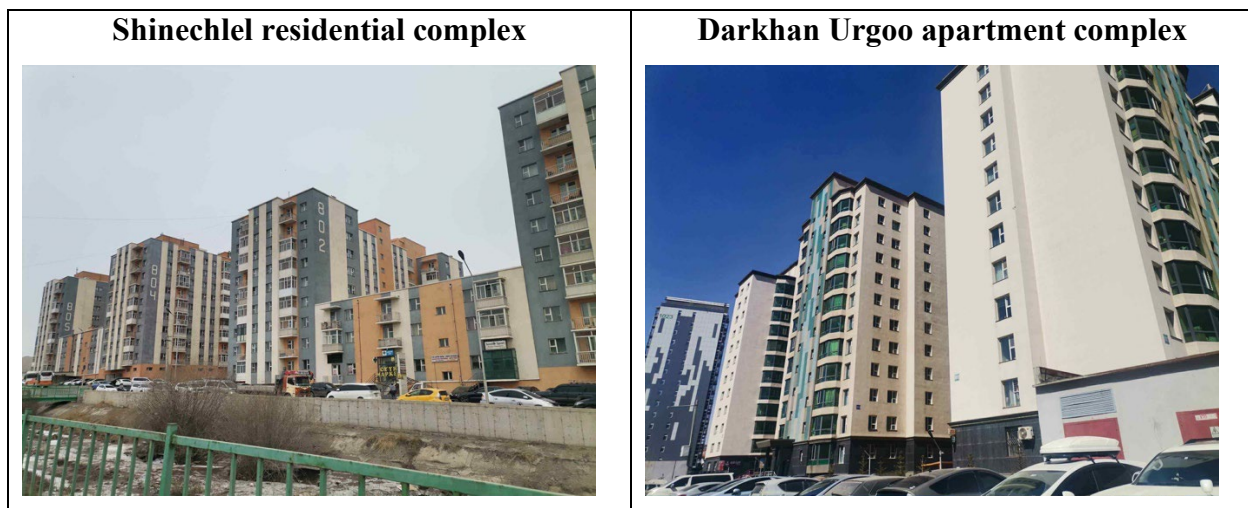
Picture 2. Redeveloped apartment buildings in two districts. Photo by the first Author, May 2025.
