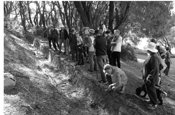
Fig. 27 Dealing with the runoff , interceptor drains on Mount Melville/Kardarup. Acting with drains, we ‘alter’ hydrology. Photo by Ian Herford
