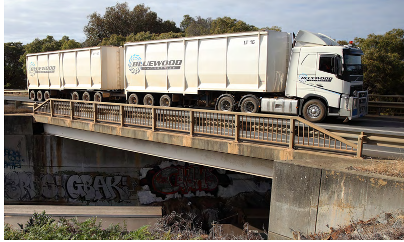
Fig. 2 Woodchip truck above and freight train below: extractivist economies in Albany. Photo © Perdita Phillips
