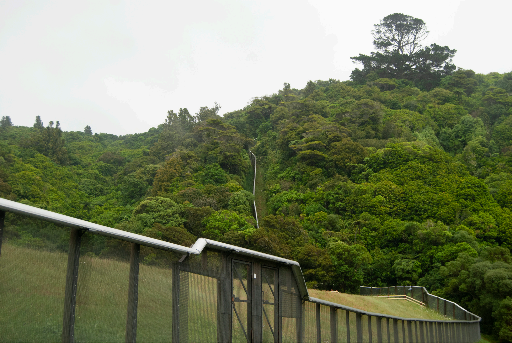
Fig. 2 Zealandia steel perimeter 'predator exclusion' fence (top) and the fence being met either side by rainforest regrowth (below). The fence is 2.2 metres high. December 8, 2019. Photos © Louise Boscacci
