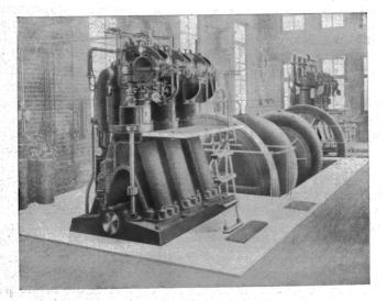
Two Diesel Engines of 120 B.H.P., each direct coupled to centrifugal pumps at the Dunedin (N.Z.) Drainage and Sewerage Board's Power House,
