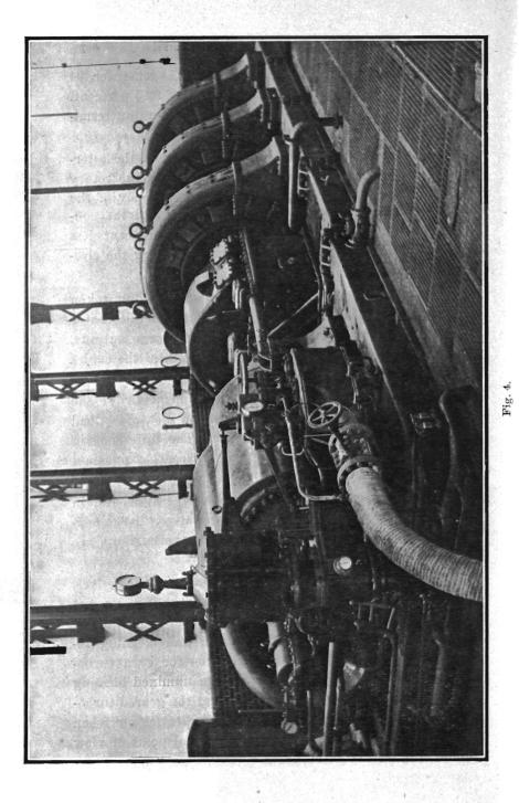
In addition to the electrical saving of 5 per cent. at full-load, and 9.5 per cent. at half-load, there is the additional saving at the steam end of the geared machine on account of a higher turbine speed being used than that synchronous to the alternator, namely, 3,000 r.p.m.
