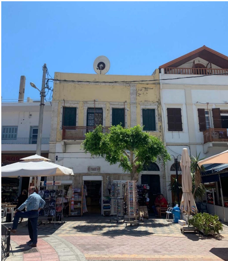
Figure 1. The 'yellow house' on Kalymnos where Clift and Johnston lived with their children. At the time, the water in the port reached up to the curved sidewalk in the bottom left corner of the photograph, where there is now a street. The shop beneath was then 'a sponge-clipping room,' but now sells, among other things, souvenirs of the island's former sponge industry.
