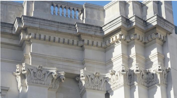
Figure 4. 'Bunches' of Corinthian entablature elements on the Sainsbury Façade.
