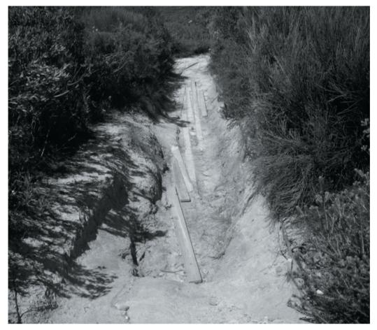
Fig. 1 An eroded and degraded sandy section of the Coast Walk, Royal National Park
