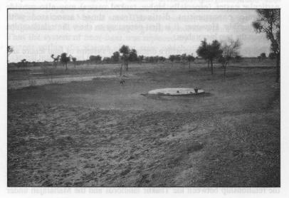
Photo 15: A private underground tank, with concave surface for collection of rainwater.
