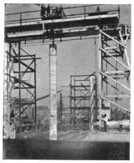
TRAVELLING GANTRY FOR HANDLING RE-INFORCED CONCRETE CYLINDERS.
