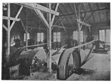
As the mine water contains CuSO, in solution, all the pipes, pump, etc., are made of brass.
