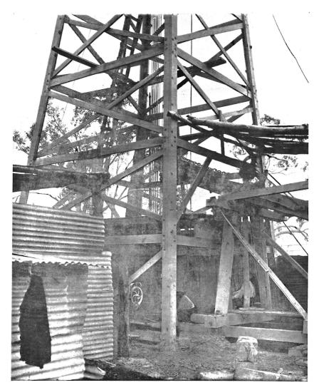
RELEASING CLAMP AND LOWERING CASING.
