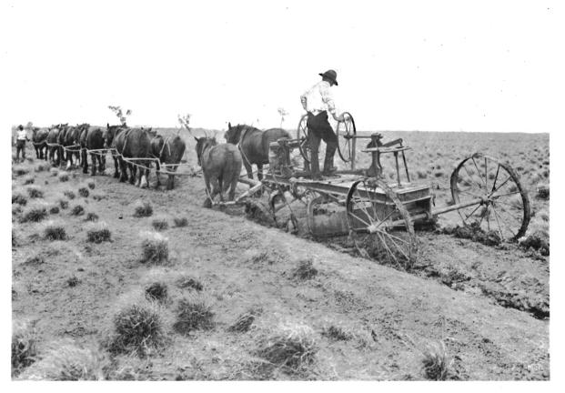
plough drawn by ten horses and weighing some 3 cwt., and to then remove the spoil with a delver drawn by some fourteen horses. The delver used by Mr. Contractor Meaney in the Moree District consists of two wings 11 feet long, formed of 2-inch planking joined at one end to form the nose, and then spread out in the form of a V 9 feet wide at
