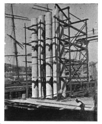
FRAMEWORK FOR ASSEMBLING RE-INFORCED CONCRETE CYLINDERS.
